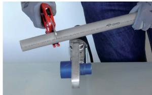
Cut the tube perpendicularly to its axis using the suitable pipe cutter.
