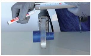
Mark the insertion depth on the pipe.
